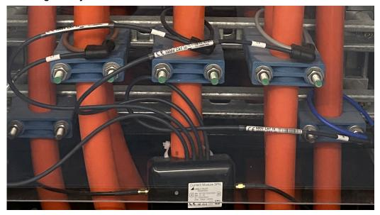
The connection housing of a current module can be fixed directly to a cable using cable ties.
