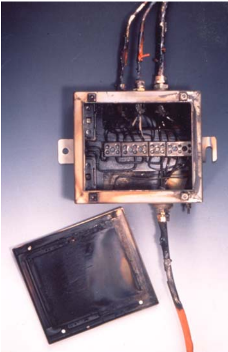
SX Range Enclosure and Cables after IEC331 Fire Testing
